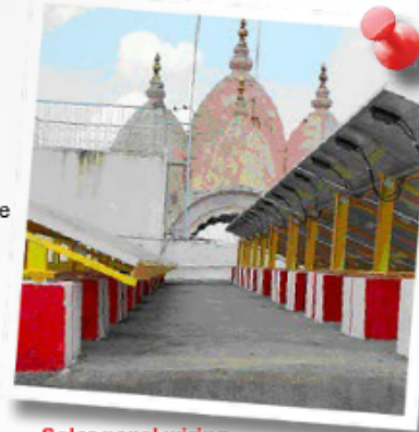
Solar panel wiring
